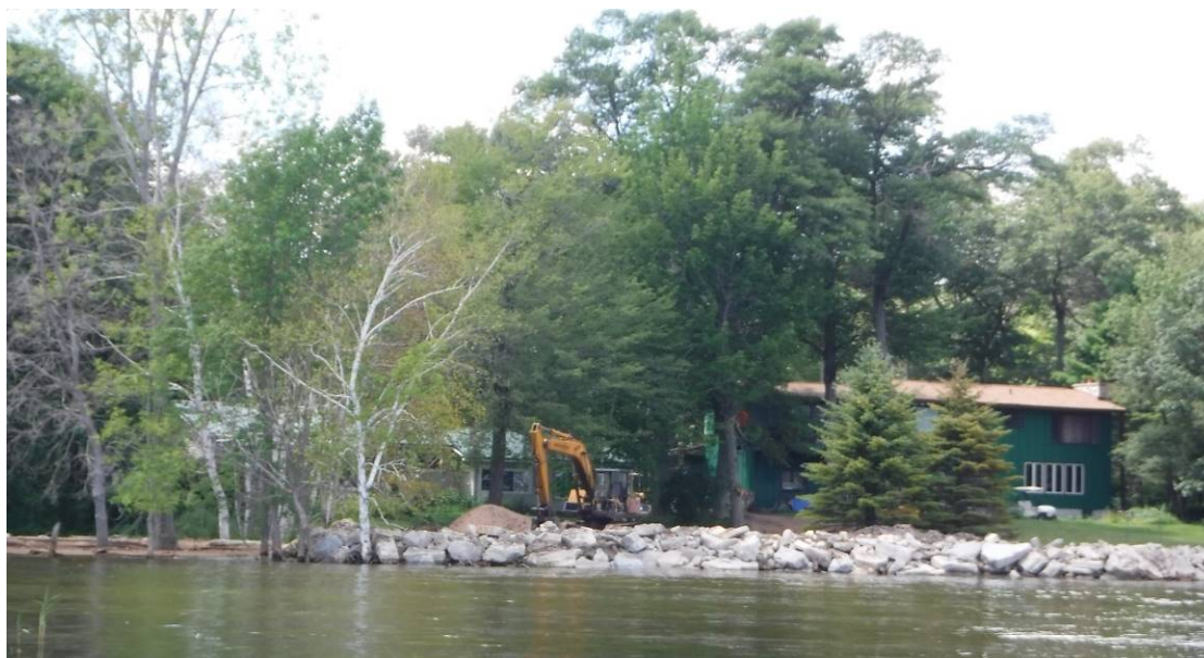
Figure 25. Several residences were adding new riprap in 2020 to protect their properties from Lake Michigan waves. Lake Michigan water levels have been increasing for several years.
